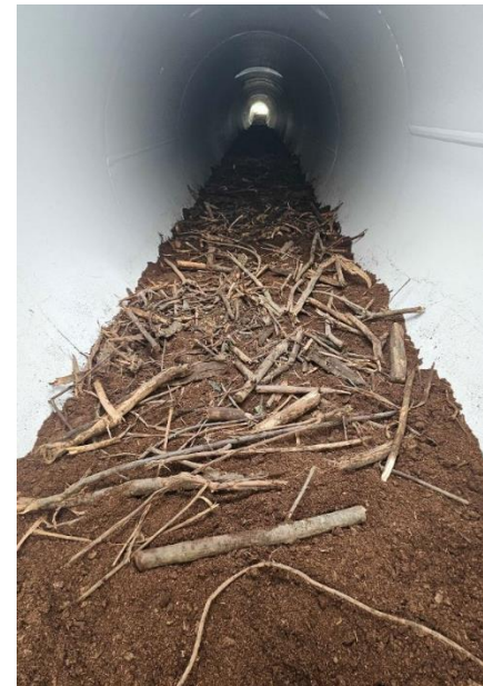
Some of the design elements include a thick layer of local, natural substrate, light boxes throughout the length of the underpass, and white reflective walls. These components help mimic the ambient environment and are known to increase the likelihood of use by wildlife.
